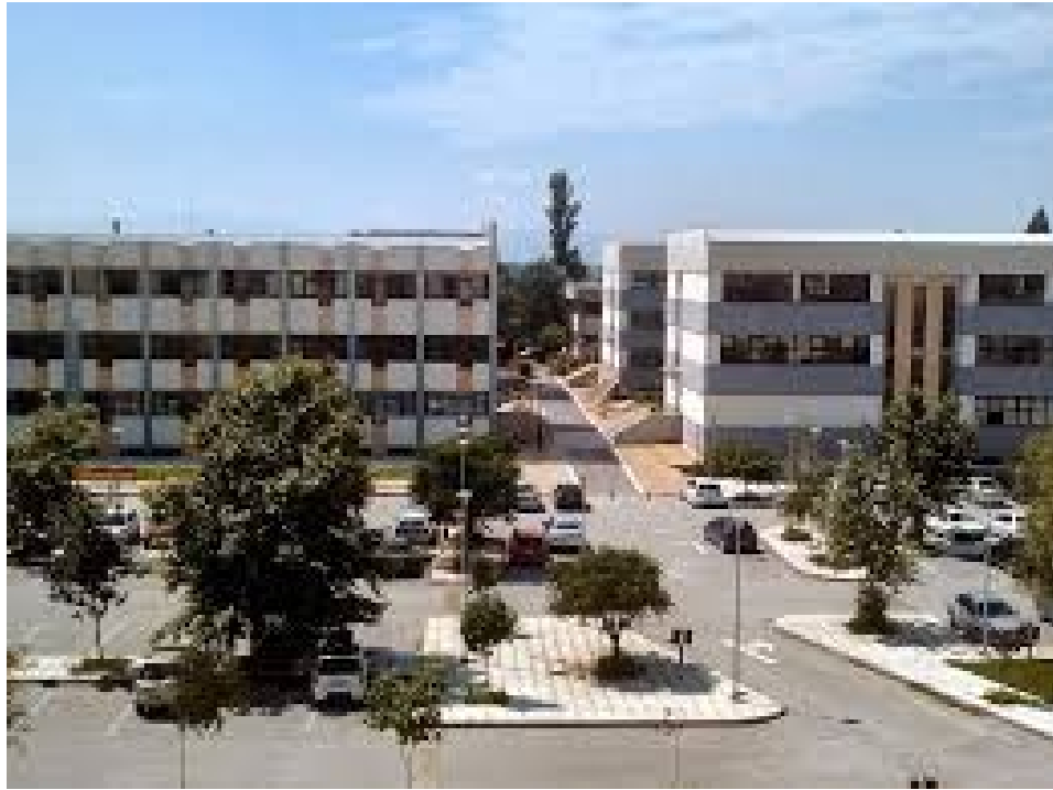
Figure 1. View of the Department's building, where Auditoriums, Clasrooms and Laboratories are located
